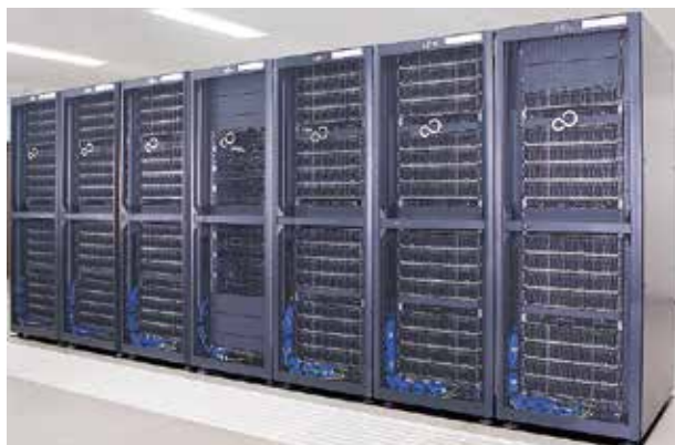
Figure 1. Fujitsu PRIMERGY CX2550.
