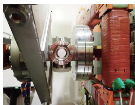
Figure 2. A new vacuum chamber for laser injection installed in the electron storage ring.
