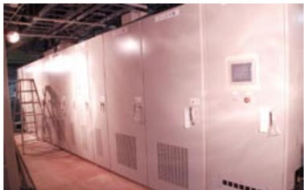
**Figure 2.** New magnet power supply for the booster synchrotron.
