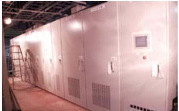
**Figure 2.** New magnet power supply for the booster synchrotron.
