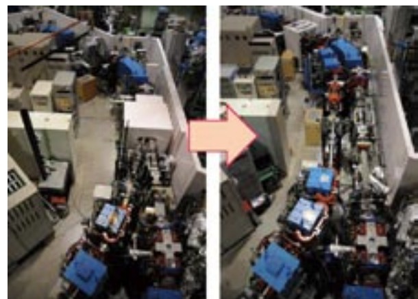
Figure 2. A part of the storage ring and the beam transport line in spring 2010, before the reconstruction (left) and after (right). The beam transport line was extended and a new 4m straight section was created in the ring. The devices colored in blue are bending magnets.
