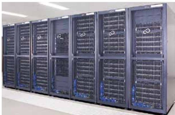
Figure 1. Fujitsu PRIMERGY CX300.
