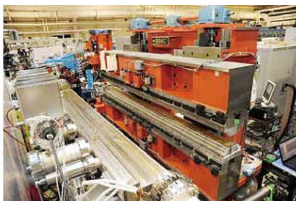
Figure 3. Remodeling of Variable Polarization Undulator at BL5U.
