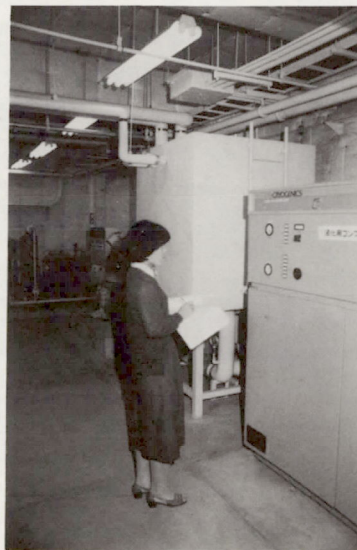
Compressors of Helium Liquefaction System
